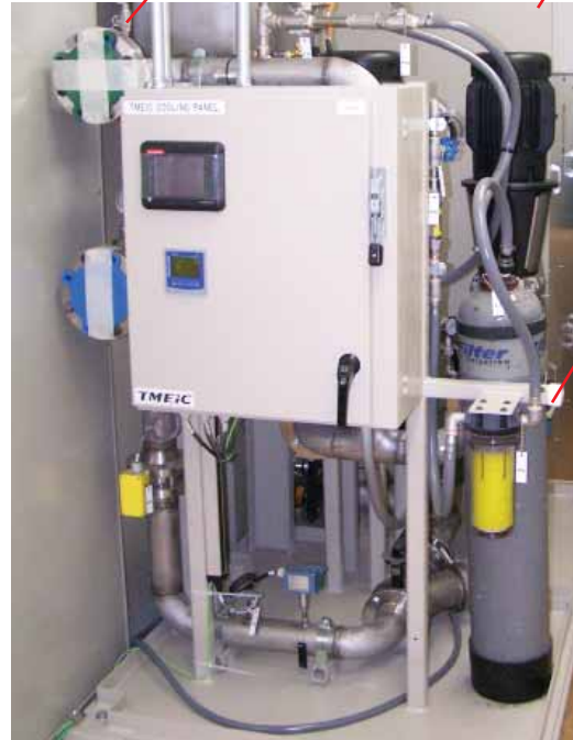
Water conditioning system behind Gate Drive Panel
