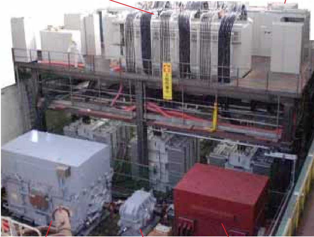
Regenerative TMdrive-70 three-level IEGT drive to recirculate power back to the supply
